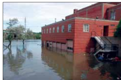
▲ The historical June flood reached Coe's Physical Plant building on the northwestern corner of the campus. As all power for the main campus is routed through that location, most of the campus was without electricity from June 12 through June 20, and the damaged electrical system went off again from July 11 through July 14.
